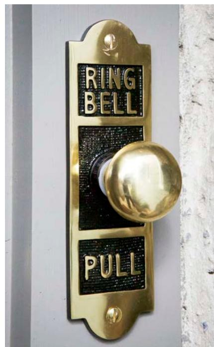
An old-fashioned mechanical doorbell hangs on the new door near the garage and rings a bell inside when the knob is pulled.
